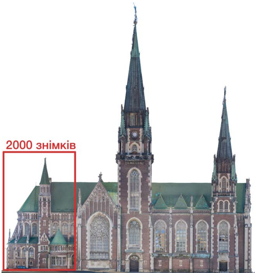
Figure 6. 2000 shots on the part of the building
